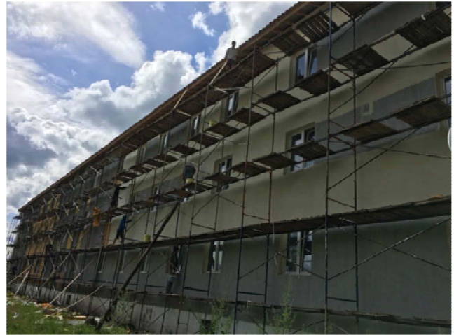
Figure 9. Finishing of the façade.
