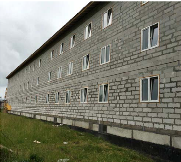
Figure 1. External walls before the insulation works.
