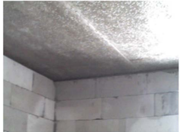
Figure 6. External wall and floor slabs conjunction zone.
