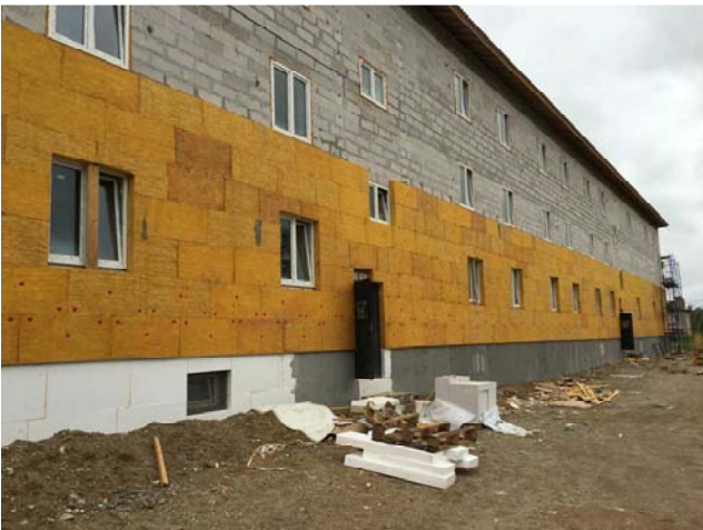
Figure 8. Heat insulation of the main façade of the building.
